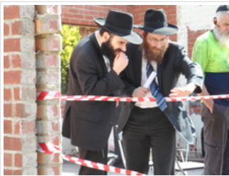
Inspecting a Mikvah in construction
